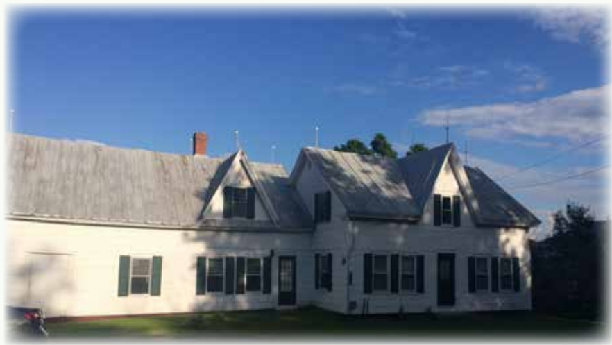
Zero Energy Now Participating Home in East Saint Johnsbury, Vermont
